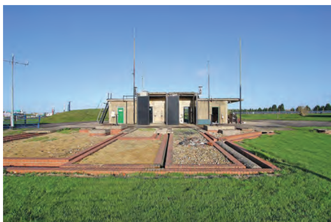
'B' Site. Note the brick-lined drainage channels in the foreground which were used to drain any surplus chemicals after motor testing
